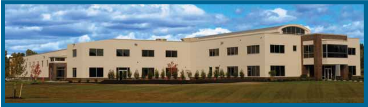
ICM Controls World Headquarters
