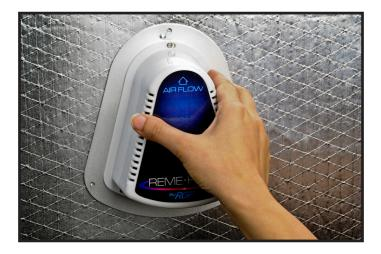
• Remove housing from unit by turning counterclockwise and pulling straight out of mounting plate.
