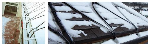
Raychem WinterGard Wet and Gardian self-regulating heating cable systems eliminate icicles and ice dams safely and efficiently.
