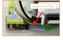
"Install the Aspen Inline filter between the AC unit's factory drain tube and the Aspen reservoir unit for ultimate protection"
