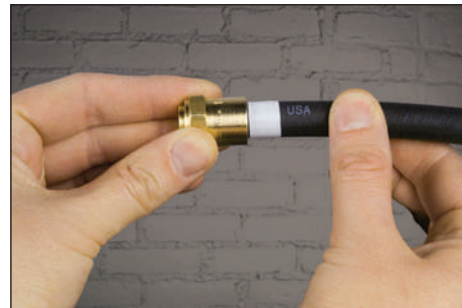
4 Verify tape line is correct for full insertion.
