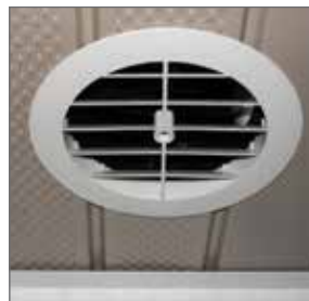
EZ Soffit Vent installed
